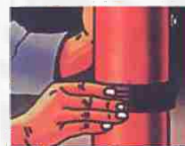
3. Next put pip or fitting on central ring and defold sealing
